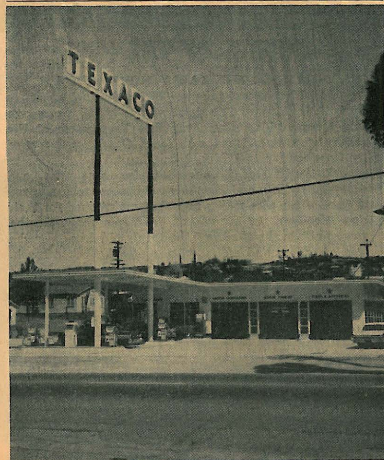
View of Bob Wilson's recently completed Texaco Service Station on Highway 80 in the center of Alpine. Echo Photo.
